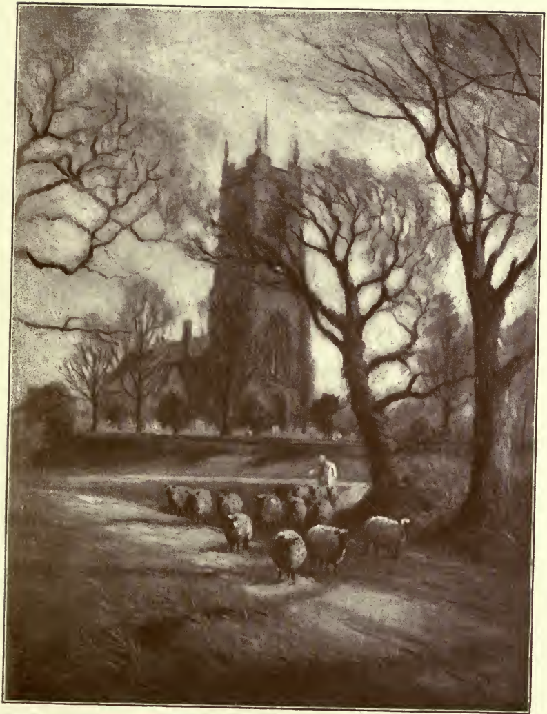
SAINT MARY'S CHURCH, DITCHINGHAM.
